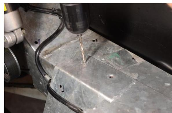
L. Insert one of the included flat-head Allen bolts through the shim and into the hole drilled in the previous step. Ensure that the large hole in the shim lines up with the threaded hole in the frame. If not, a larger may be in order.
